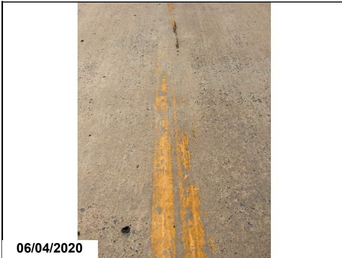
Unsealed cracks to deck.
