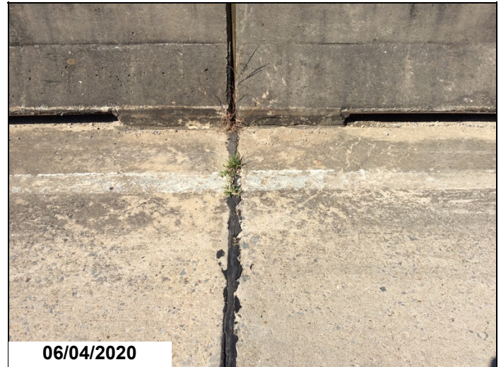
Typical deck cracking on Left & Right edges of deck over Bents.
