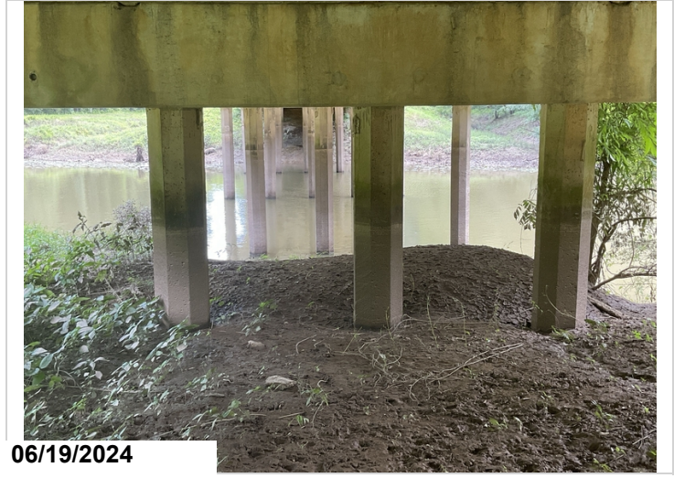
Piles: Minor abrasion throughout the structure.
