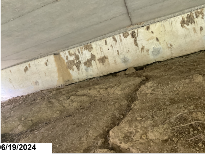
Abutment 2: Minor erosion causing one pile to be exposed.
