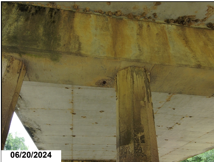
Spalls to cap with rebar exposed to Bents 2 & 3. Bent 3.
