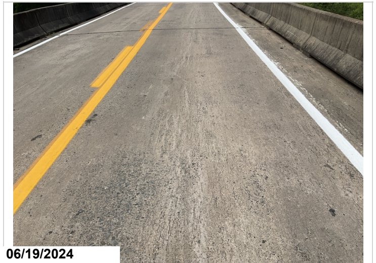
Spans 1 - 5: Minor abrasion.
