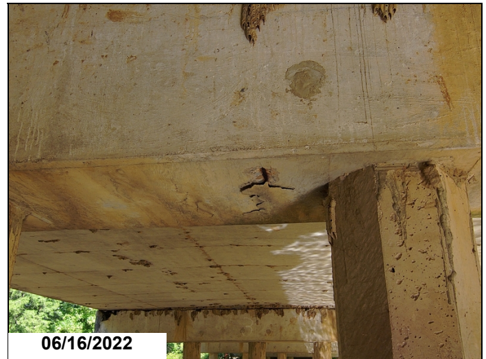
Spalls to cap with rebar exposed to Bents 2 & 3. Bottom of cap between piles 3 & 4 @ bent 3.
